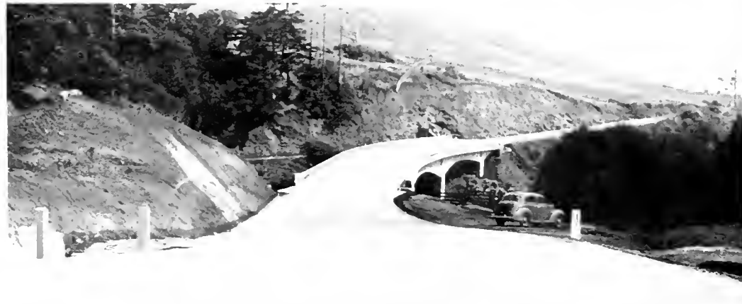
Curvature of structure conforms to 300-foot radius center line
